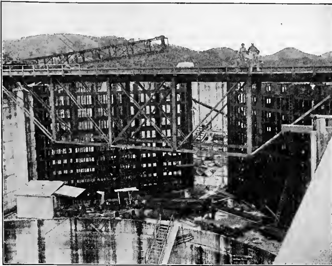
BUILDING AN UPPER TIER OF LOCKS
